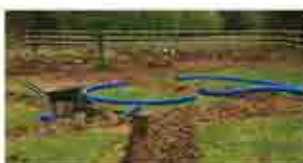
Groundworks & Land Drainage
