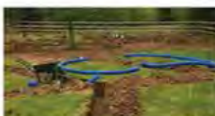
Groundworks & Land Drainage
