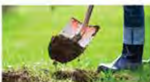
Planting & Irrigation Work
